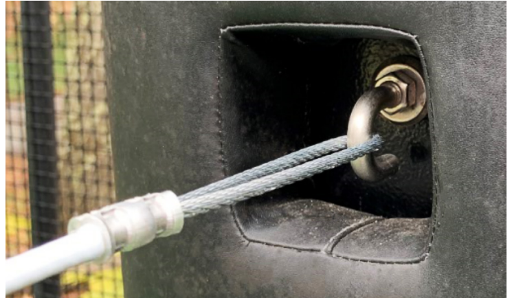
Figure 3: One end of net cable attached to the basketball/fixed pole.
